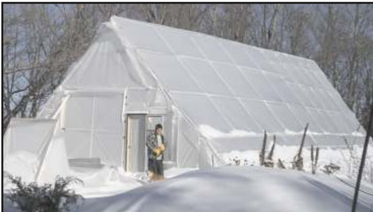
Bob in front of our 2006/2007 A-frame. Bob soon had to go inside because of the wind-chill factor outside that day. (The tiny A-frame in front is a movable cold frame for seasonal protection of outdoor plants in spring and fall.) The big A-frame is 35 ft x 60 ft x 18 ft tall. Note how the snow slides off without assistance from us. The Poly at front top needs to be trimmed off when the weather warms up again.
